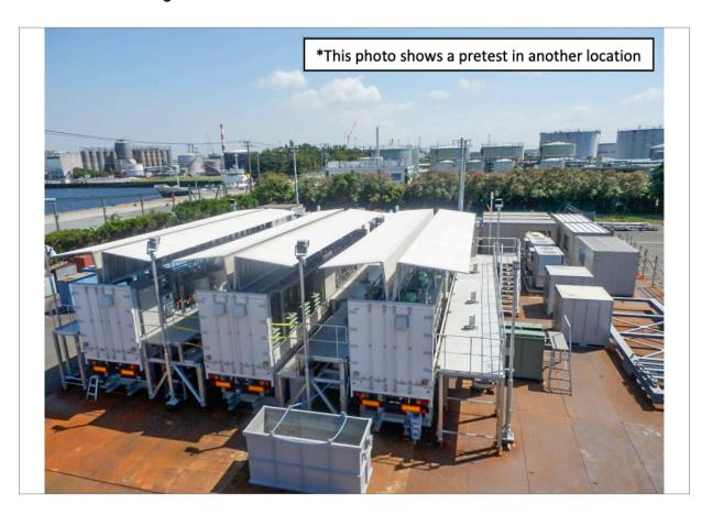
The facility for the treatment of radioactively contaminated oil/water mixtures has now been successfully put into operation in **FUKUSHIMA DAIICHI**. Diamond electrodes from **DiaCCon** take over the cleaning process (advanced oxidation).
